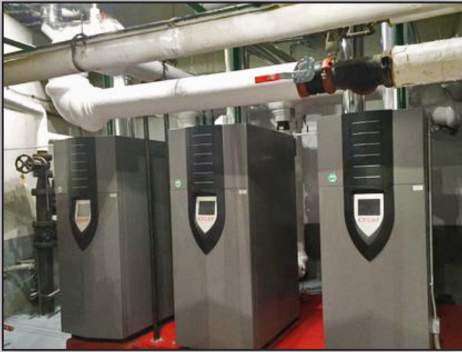
3 FBN-2000 Crest Condensing Boilers replace the 2 million Btu/hr cast iron boilers
